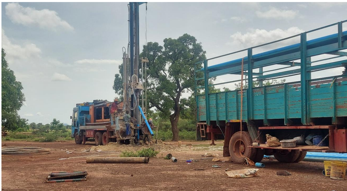
Photo 1. Drilling operation in Toéga (09/07/2025).
